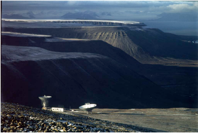
Figure 5: Overview of the EISCAT ESR site on Spitzbergen. KAMFAB 32-m antenna to the left, Alcatel fixed 42-m antenna in the foreground.
