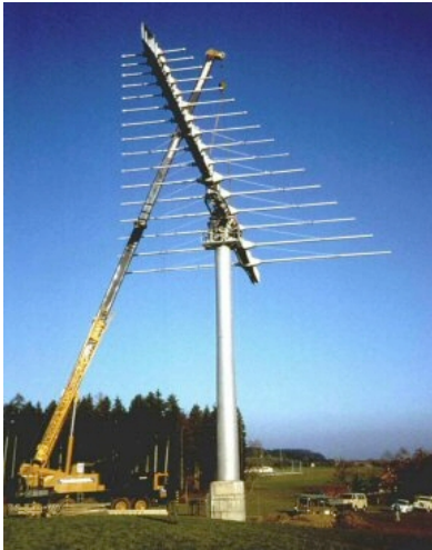
Figure 7. An Allgon log-periodic antenna in Switzerland.
