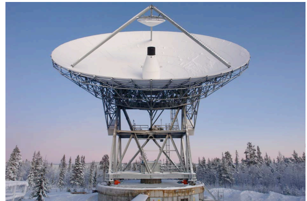
Figure 1: The Kiruna EISCAT UHF antenna in Cassegrain configuration
