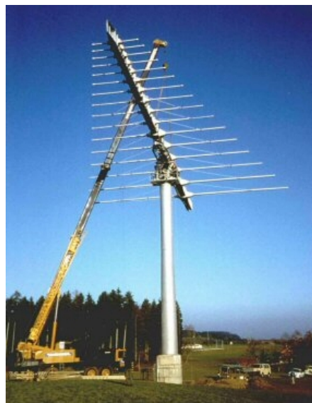
Figure 3. An Allgon LPD16 antenna during its dismantling in Switzerland. The Allgon LPD 16 K was a steerable logperiodic antenna for communication over medium and long distances in the HF range. It was designed for transmitters up to 250kW per carrier and 100% AM modulation over the entire frequency range 6-30MHz. The boom was tiltable allowing for beam shaping to optimize the communication.
