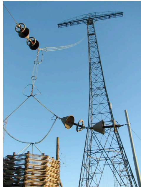
Figure 2. One antenna tower with the cage type vertical radiator and tuning coil visible (Wikimedia Commons).
