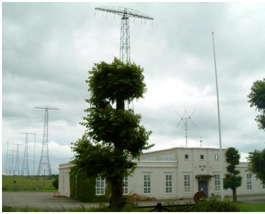
Figure 9. The Grimeton station building and the six antenna towers (Wikimedia Commons).
