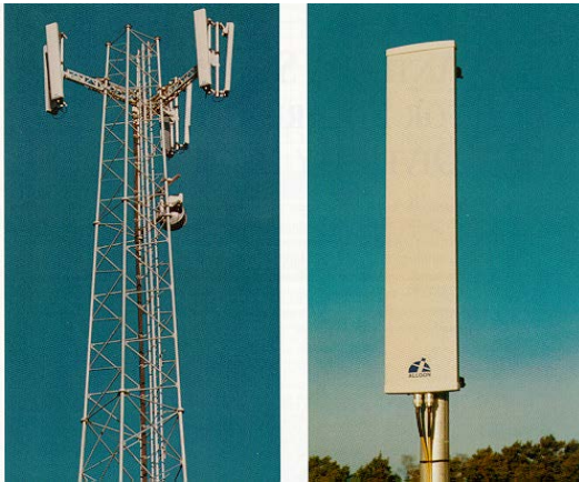
Figure 5. Base station antennas for GSM: a) in a space diversity configuration b) using polarization diversity which dramatically reduced the space and windload for the same performance
