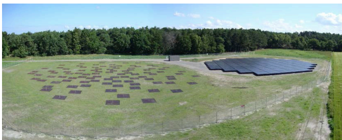
Figure 3. The LOFAR station at Onsala (OSO).
