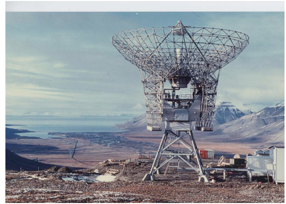
Figure 4: The KAMFAB ESR Antenna just before installation of reflector panels. Summer 1995.
